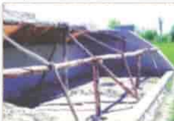
Picture No. 14: Adjusted skeleton for fixation of the polythene sheet
