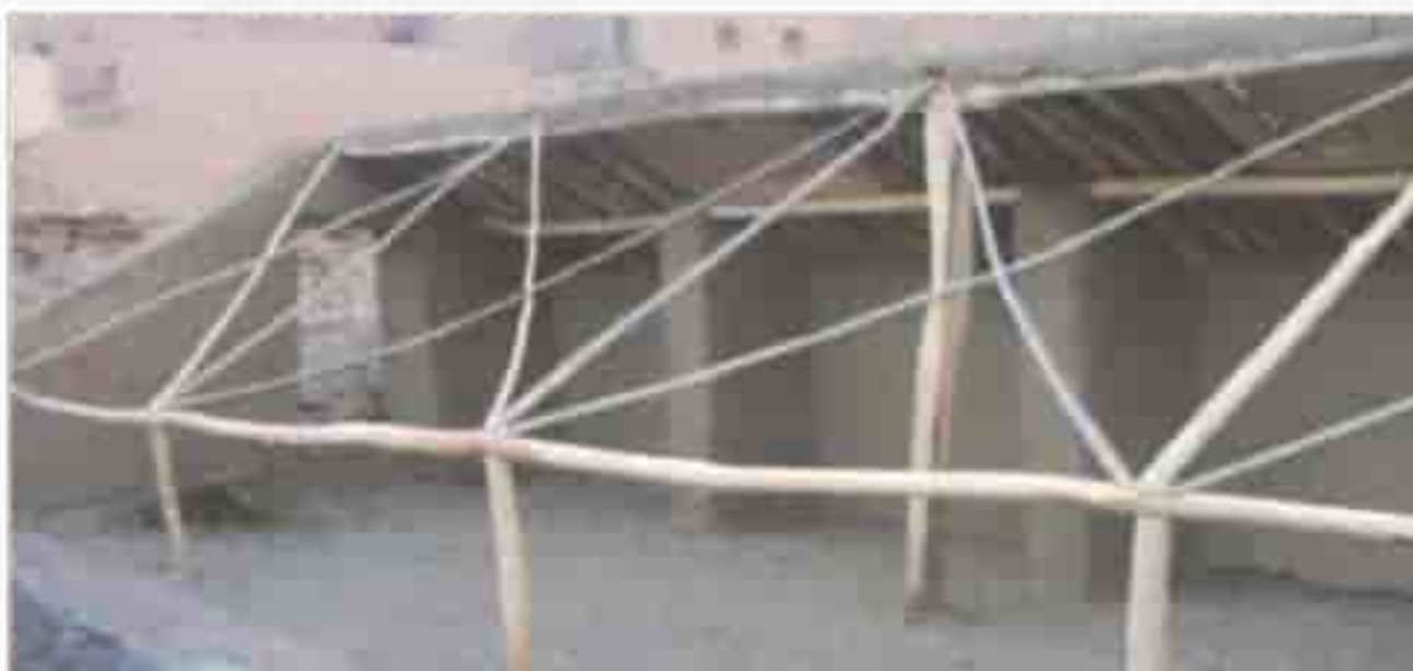
Picture No. 10: The inner construction of the greenhouse – main horizontal beam supported by wooden slope and the second horizontal beam supported by the partition north walls.
