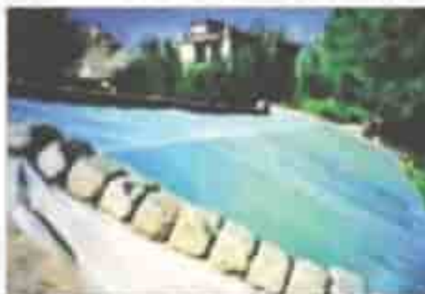
Picture No. 15: Top and side fixation of the polythene sheet by the mud layer and mud bricks
