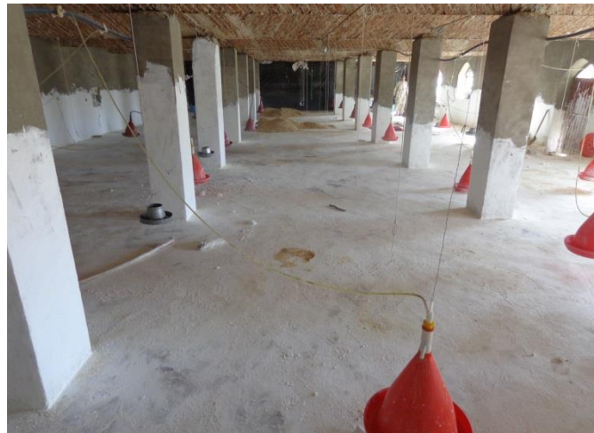
A room painted with lime after cleaning.
