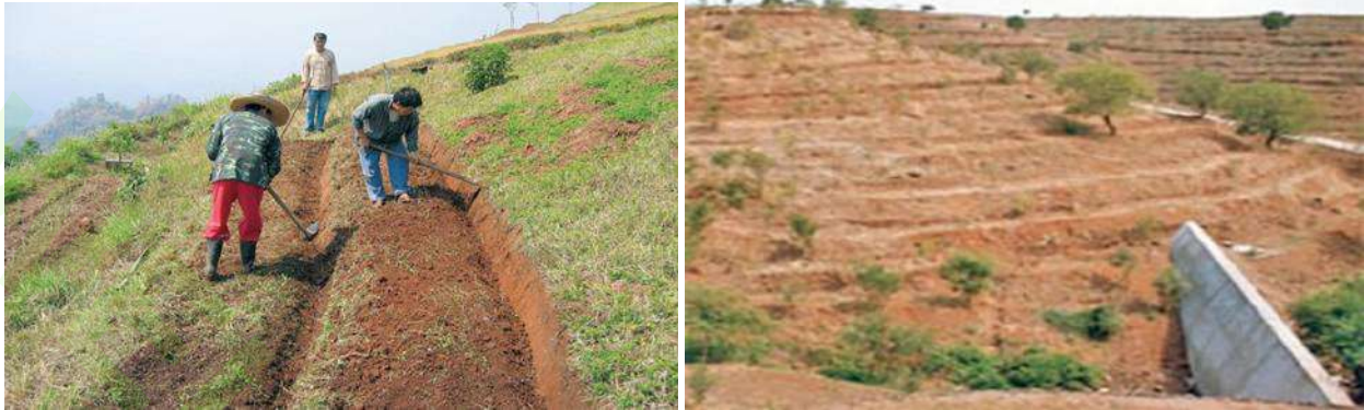
Figure 9 and Figure 10: Contour bench terraces
